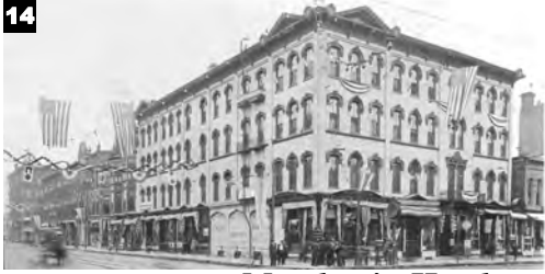
Northeast corner of 4 th and Pierce Street
