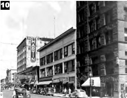
North side of the street between Nebraska and Pierce Streets (515-521 4 th Street)
