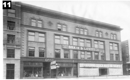
South side of the street between Nebraska and Pierce Streets (514-520 4 th Street)
